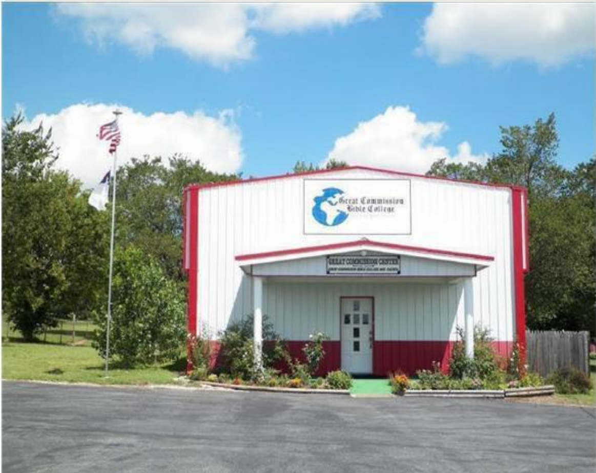
Photo above is GCBC Administration Building
